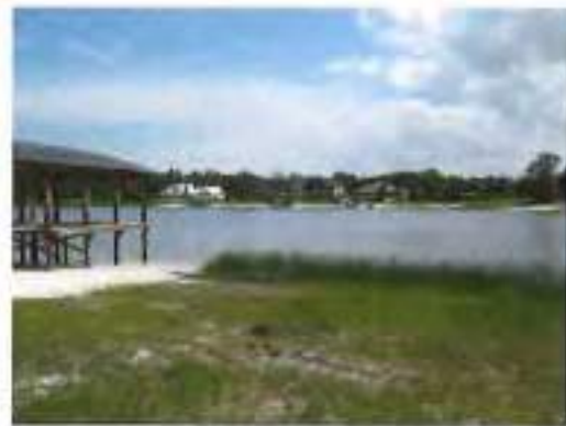
Figure 9. Shore erosion in Lake Mary
